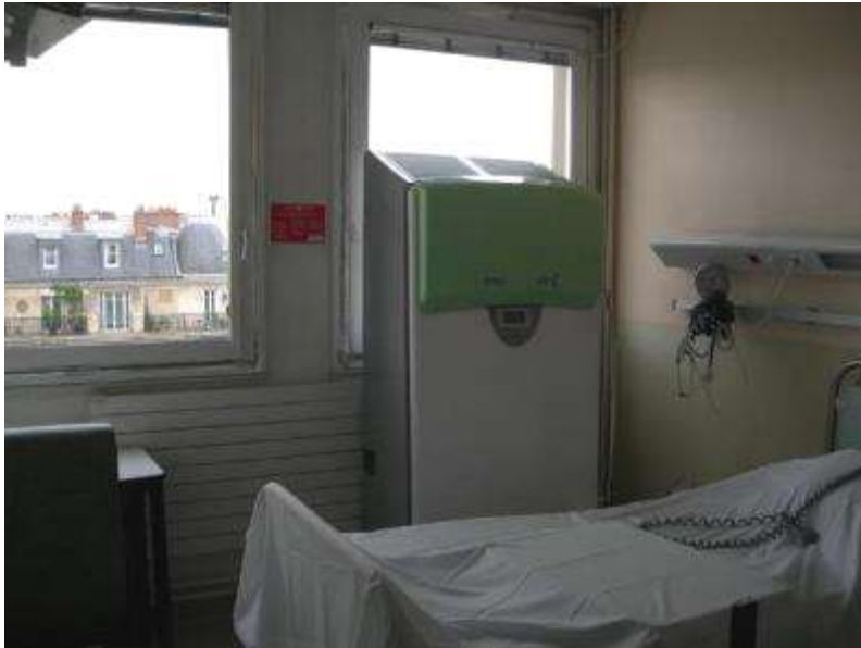
Hematology – Autologous BMT Patient room 55 m 3 PA-T2006NG – 1,000 m 3 /h ISO9=> ISO7 in less than 10 min
