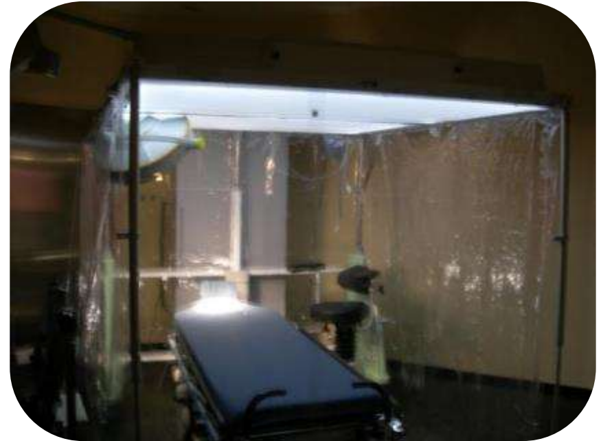
Hematology – Allogenic BMT Patient room IMMUNAIR w/T2006NG– 1100 m 3 /h ISO9 => ISO5 in less than 6 min
